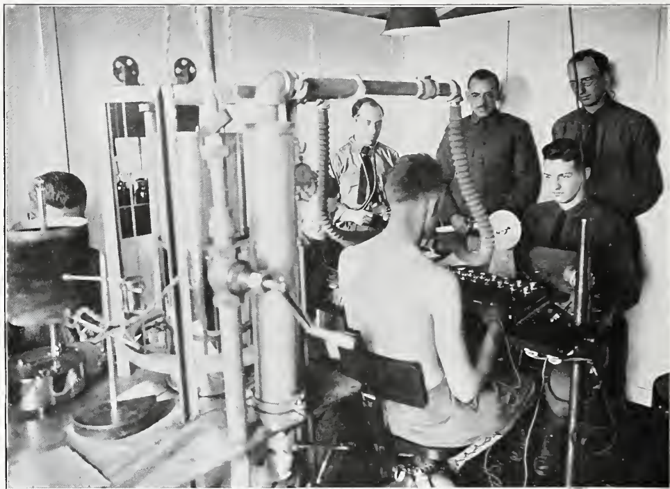
FIG. 136.—Low oxygen tension test room, aviation hospital.
